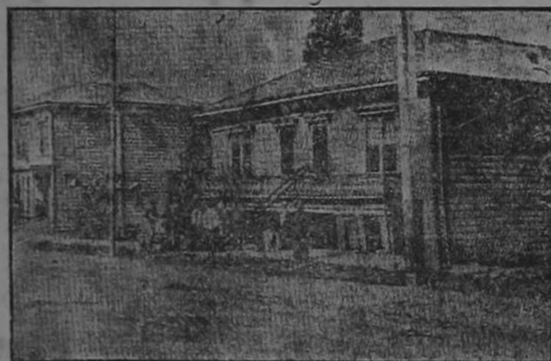
HOUSE SUNK WHEN GROUND OPENED IN EARTHQUAKE.
